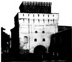
Fig. 14.2. The Vlassyevskaya, or Znamenskaya tower that had formerly been part of Yaroslavl’s sturdy fortifications, destroyed in the Novgorod pogrom (according to our reconstruction). A view from the west. Modern photograph. Reproduced in accordance with [1996], page 73. In the left corner of the Znamenskaya Tower one can clearly see the remnants of a brick wall, which had once stood adjacent to the tower. The wall was destroyed – there is nothing left but uneven marks.
